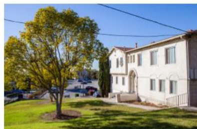
Campbell Hall exterior
